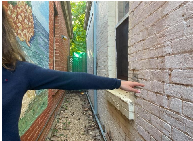
Southern wall of 114 Sydenham on right side of photos showing windows & metal poles supporting crooked wall.
