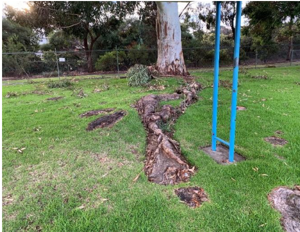
Tree 2. Large, exposed surface roots present as a trip hazard.
