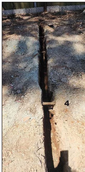
Very few roots encountered 1>50mmØ. New species Water pipei discovered.
