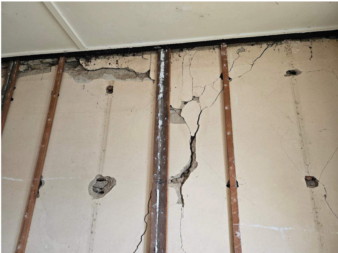
Photo 4 – Bed 1's northern wall
