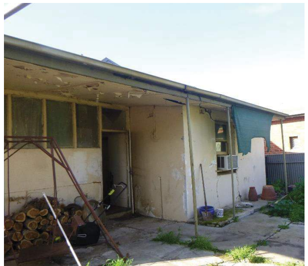
Lean-to construction at rear
