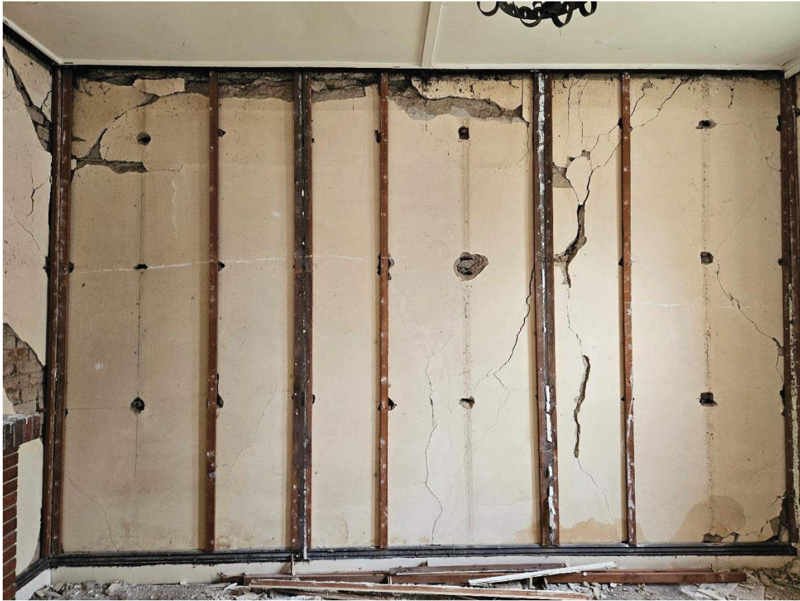
Photo 3 – Bed 1's northern wall
