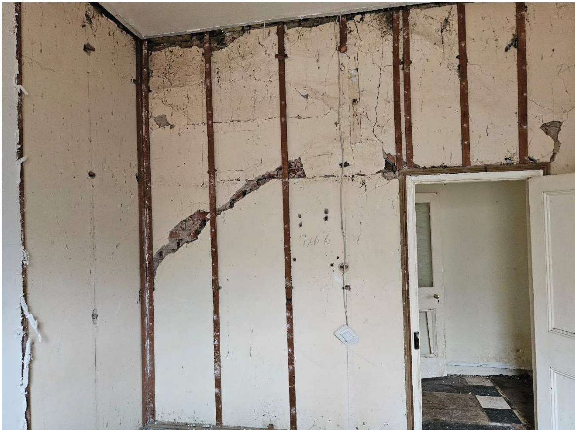
Photo 14 – Overall view of living room's northern wall
