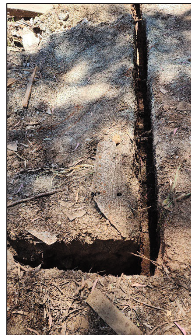
Trench extended to west given proximity to tree
