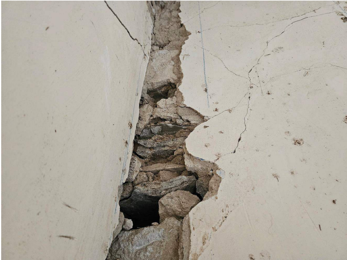
Photo 11 – Internal view of external wall showing random stone masonry construction
