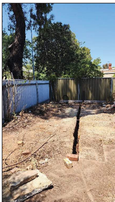
7.6 mtr long x 800 mm deep hydrovaccated trench completed.
