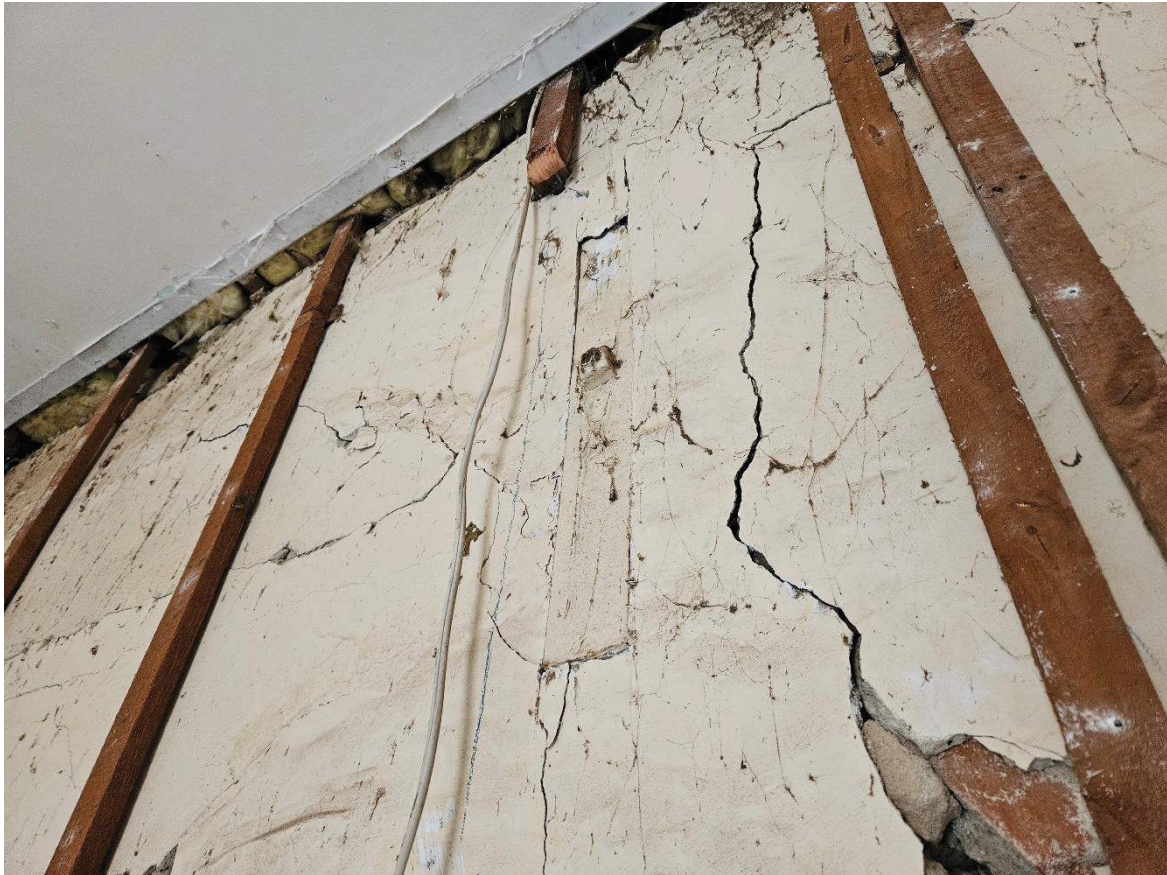
Photo 15 – Tie rod end plate in Living room's northern wall, rotation of brickwork around end plate
