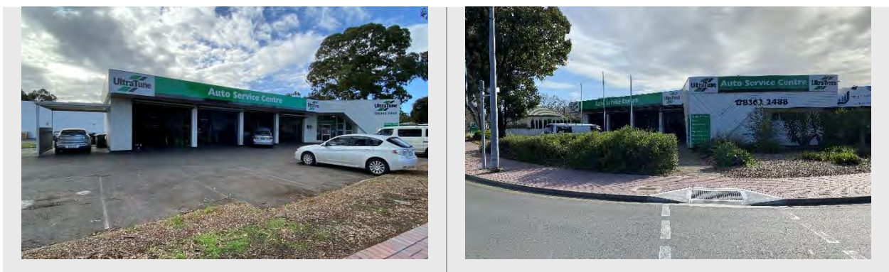
Existing building from Stephen Terrace looking east
