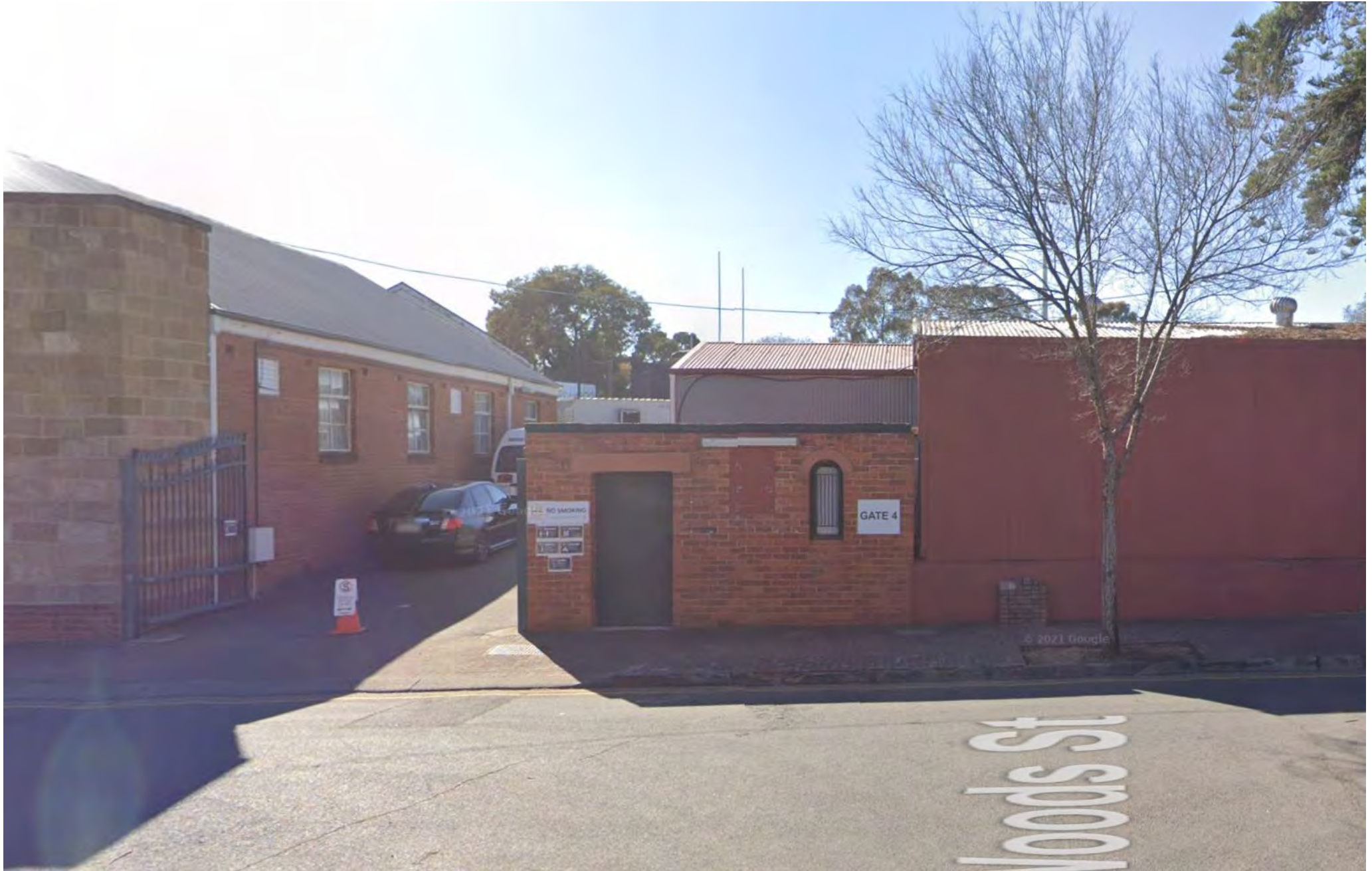
EXISTING TICKET BOOTH
