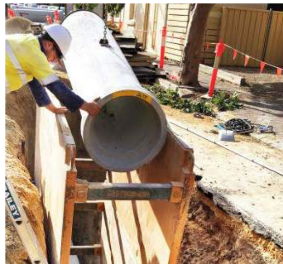
Stormwater infrastructure upgrades
