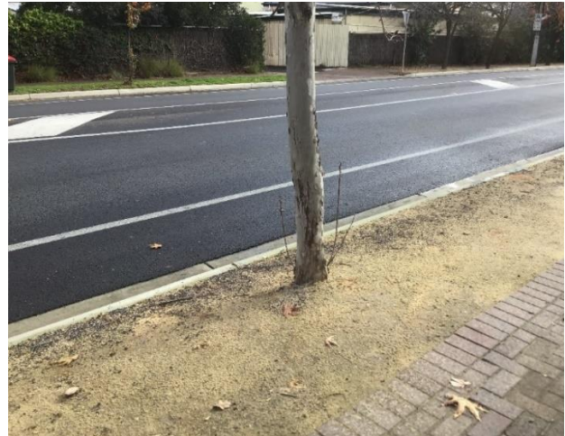
Quartzite - Stephen Terrace, St Peters (Note proximity of quartzite to young tree)
