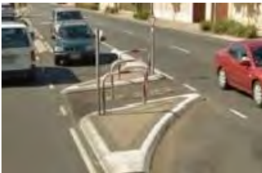
Figure 4 Example of Cyclist Central Median Refuge Island
